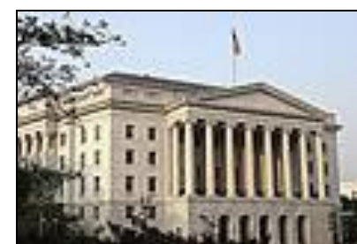
Longworth House Office Building
